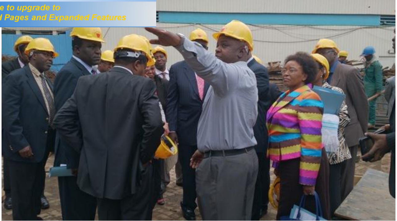
Members of University of Nairobi top Management led by Vice-Chancellor, Prof. George Magoha, carry out a site inspection of University of Nairobi Towers.
